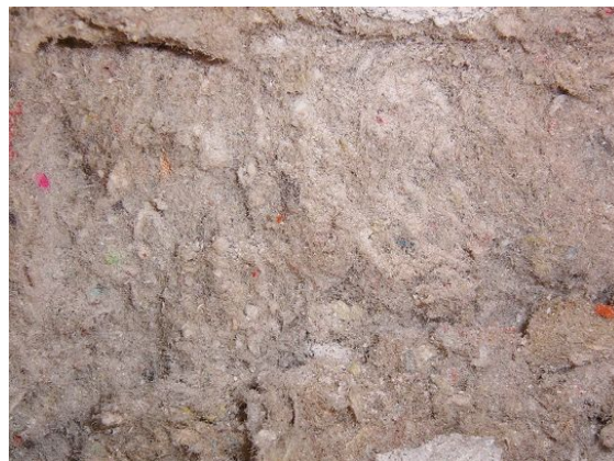
Figur 6.4.2 Papirisolering i hulrum
