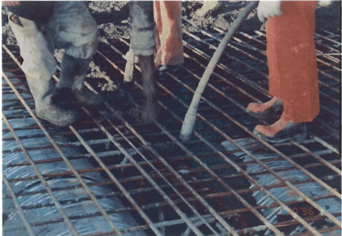
Fig. 19. Casting of prestressed slab with corrugated cavity tubes.
