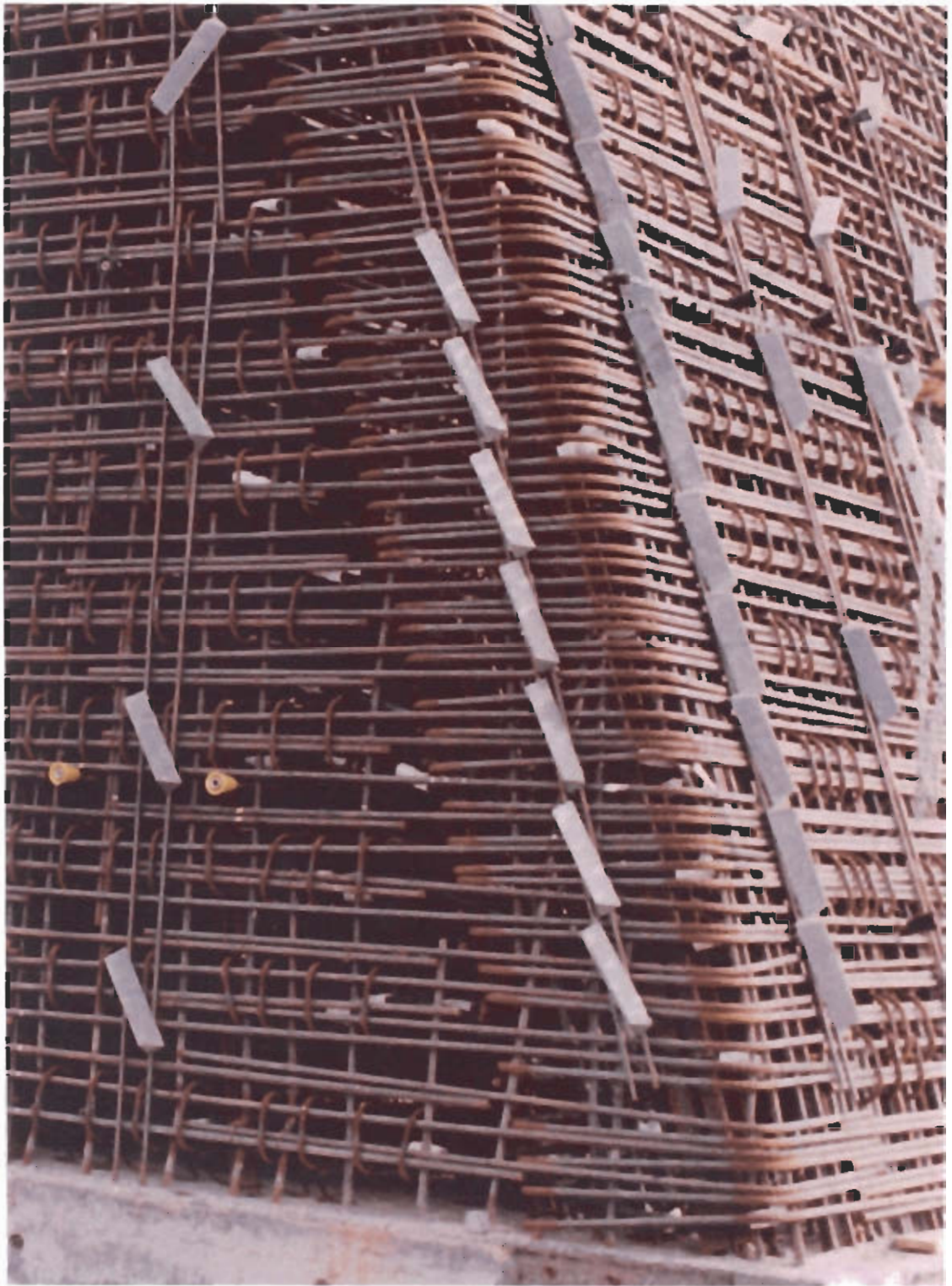
Fig. 30. Closely spaced anchored bars
