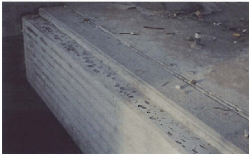
Fig. 15. Recess with holes from rising air bubbles.
