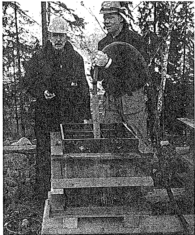
Fig. 11 — Testing in special forms was carried out to determine the influence of vibrator insertion on frost resistance.
