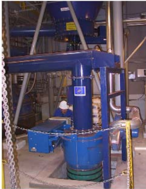
The bottom of the ash silo, the new screw conveyor and the load bellows at AWS.
