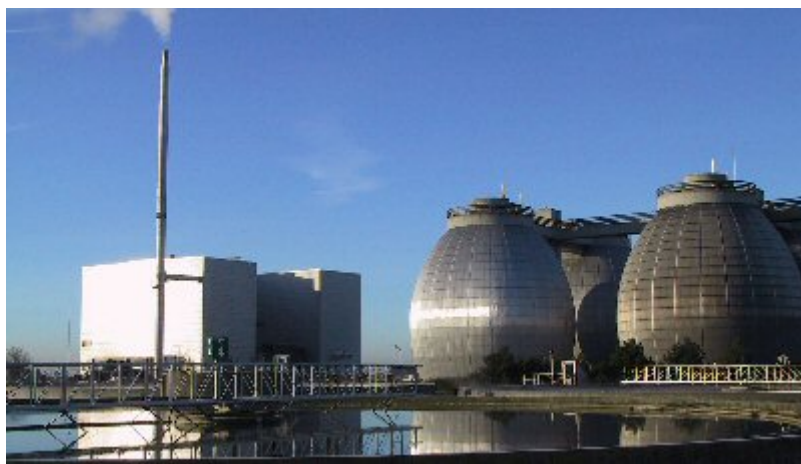
Waste Water Treatment Plant, Avedøre
