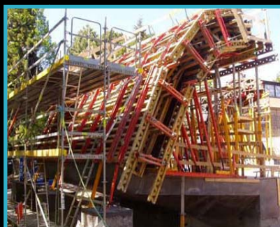
Example of expensive manual construction process, instead robot manufactured formwork could have been used with advantages.
