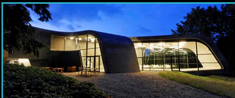
Tomorrow's unique concrete structure. Displayed is the addition to the Ordrupgaard museum constructed in 2005.
