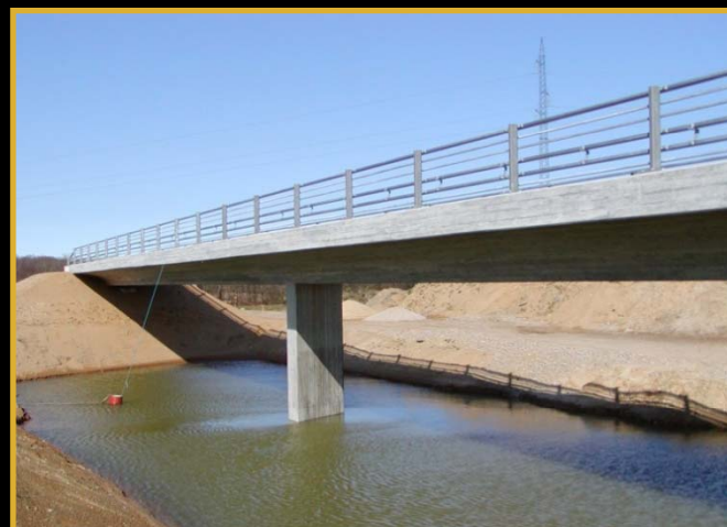
Highway bridge in Western Denmark cast using only self compacting concrete.
