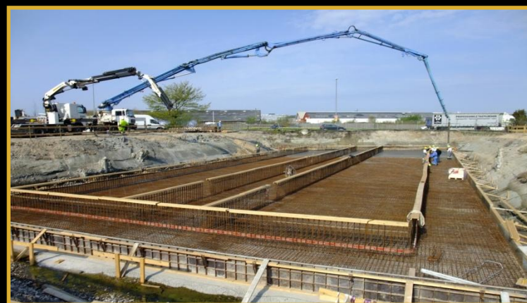
The bassin slab is 900m 2 in total and 40cm thick. Reinforcement needed to withstand high water pressure from underneath, due to a high groundwater table. Due to the use of SFRSCC a lot less steel had to be placed manually which in itself is a clear cut bonus for the working environment.
