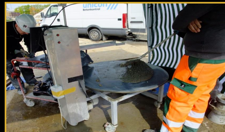
Target slump flow for the mix design was 550mm. Strict control of the concrete rheology and slump flow was kept using the 4C-Rheometer. Slump flow below 500mm made the SFRSCC very difficult to place and slump flows higher than 600mm made the concrete front more difficult to control and increased the risk of segregation.
