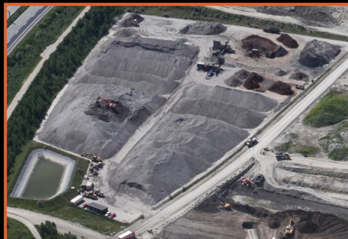
One of four danish AFATEK storage facilities for bottom ash. Processing and removal of metals is performed locally.
