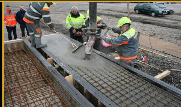
Trial castings were carried out to optimise the flow properties and casting procedure. By using SFRSCC the total amount of steel could be reduced. Right: Beam with 16mm rebars and no fibers. Left: Beam with 10mm rebars and 30kgs RC-80/60 BN steel fibres.
