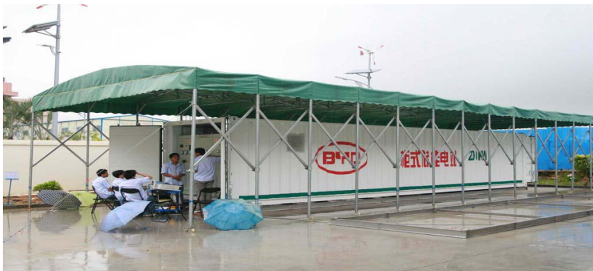
Figure 3.1.9: BYD 800kWh / 200 kW container for bulk storage
