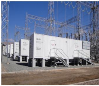
Figure 3.1.5: From A123 Chile installation
