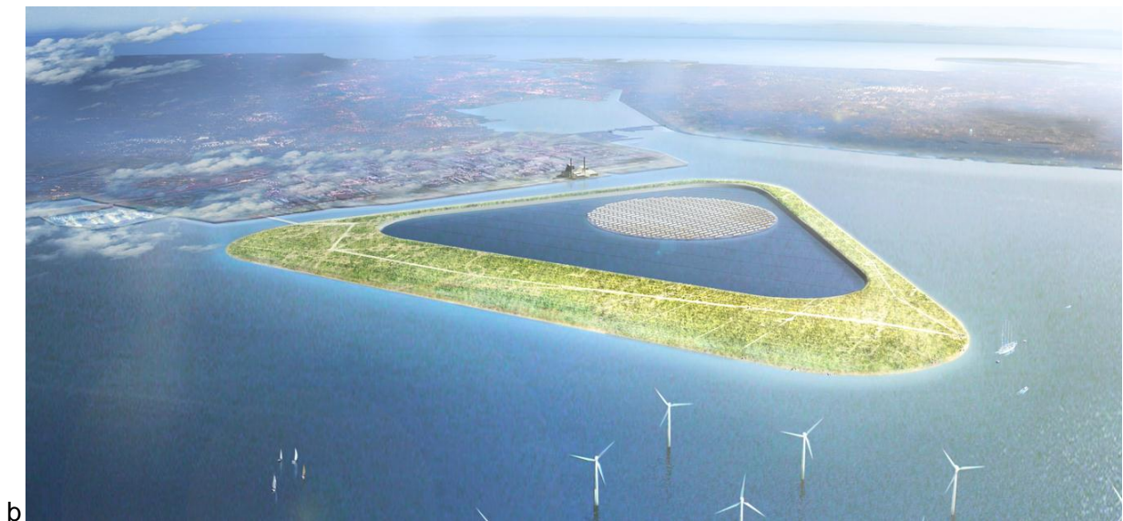
Figure 3.4.2. Artistic drawing of an Energy Island 26 . Water from the deep interior of the island is pumped out in periods of surplus electricity. The electricity can subsequently be regenerated when water is allowed to flow back via turbines. The concept may be expanded with wind turbines (on-shore foundations), solar cells (circle in the middle) as well as algae production.
