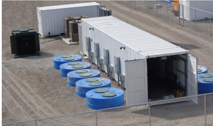
Figure 3.3.3. Photo of Beacon Power flywheel installation in commercial operation in ISO New England, USA, since November 2008. The picture shows 10 flywheel modules lowered into the ground (5 on each side of the container). Source: Beacon Power.
