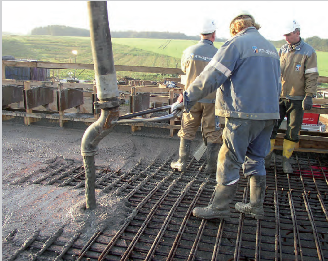
Figure 2.5. Pumping SCC for horizontal applications. The pump attendant controls the outlet of the pump hose while a pump operator controls the pump itself and the pump pressure.
