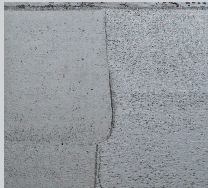
Figure 4.7. Upper left: Throwing of SCC floor slab. Knowing the right time to carry out trowelling is a matter of experience. Particularly for larger floor areas it is important to pay attention to the uniformity of the flow properties of each batch. Otherwise it will cause non-uniform surface quality that makes it difficult to perform trowelling. Upper right: SCC bridge deck surface finished with a surface planer (left) and a drainpipe tool (right). The slump flow is approximately 480 mm and the viscosity is relatively high. The planer leaves visible tracks from aggregates while the drainpipe tool has a difficult time submerging the aggregates. Bottom right: Examples of different surface finish procedures applied on the same floor – trowelled, grinded and a broomed surface.
