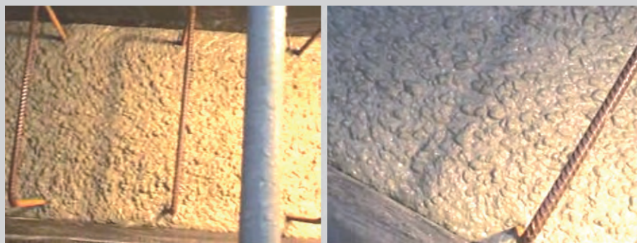
Figure 2.9. No segregation (clearly visible aggregates on the surface) – A rough construction joint can be established.
