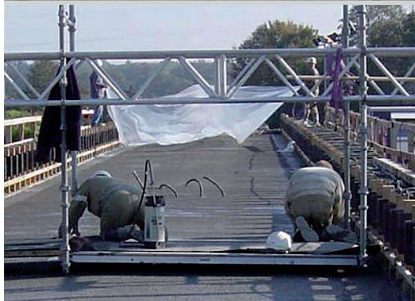
Figure 2.15. Top: Plastic shrinkage of a concrete floor. Bottom: Application of plastic covering on SCC bridge deck.
