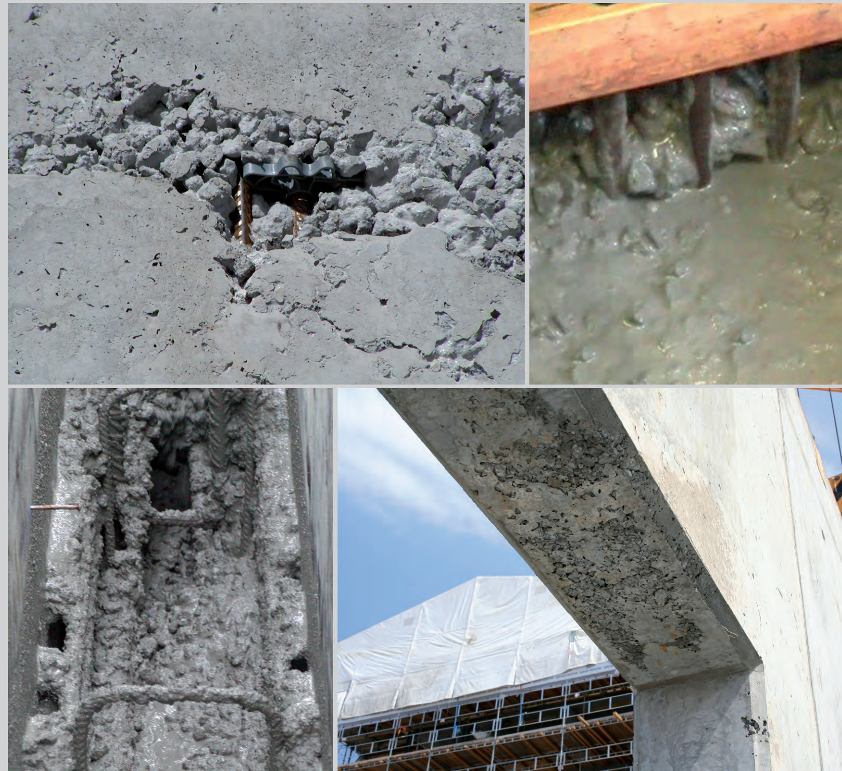
Figure 2.12. Blocking during SCC castings. Examples of congested reinforcement and accumulation of aggregates behind the reinforcement and honeycombing.
