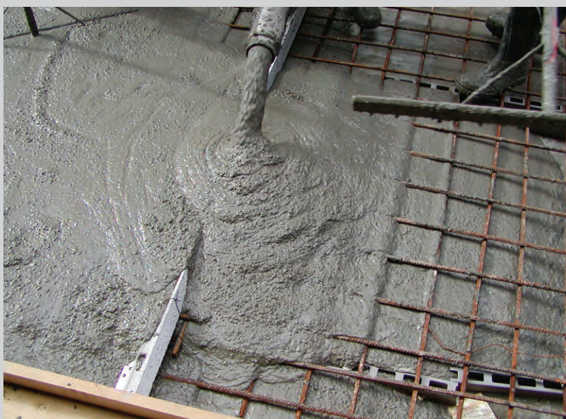
Figure 4.5. Left: Horizontal casting of SCC. Right: SCC is placed using a scraper so that the concrete is redistributed in order to obtain correct slab thickness.
