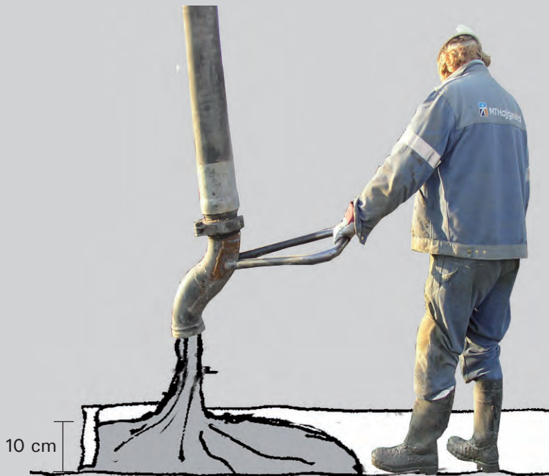
Figure 4.3. Example of floor casting with a low slump flow value of approximately 525 mm. Good control of the concrete front where it is easy to reach the final concrete slab depth (e.g. 100 mm) during a single filling process.
