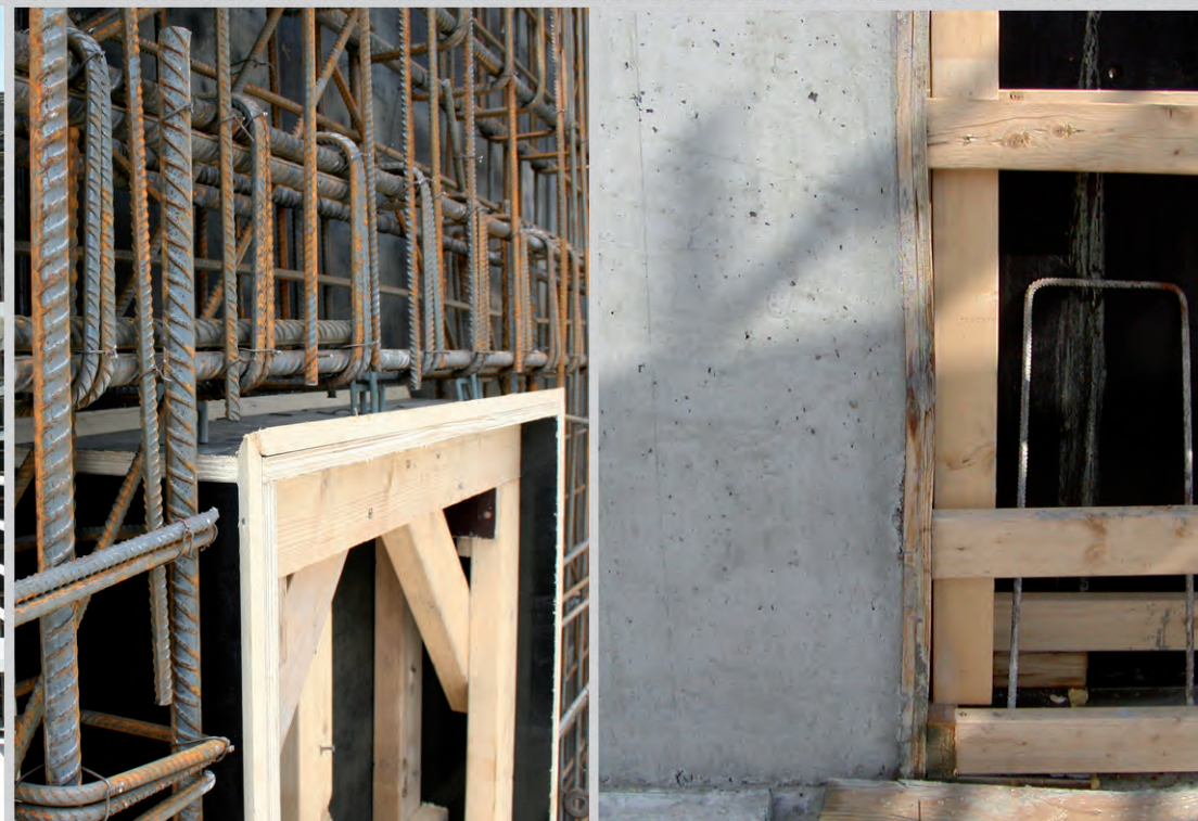
Figure 2.3. Preparations of wall formwork with a height of approximately 4 m. Example of recesses and box outs.
