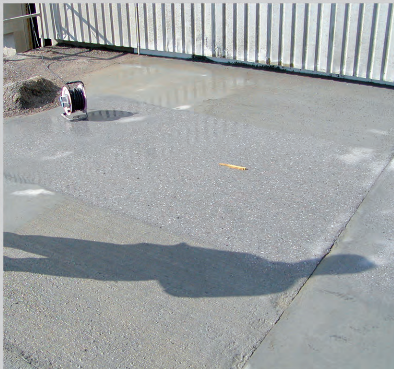
Figure 4.7. Upper left: Throwing of SCC floor slab. Knowing the right time to carry out trowelling is a matter of experience. Particularly for larger floor areas it is important to pay attention to the uniformity of the flow properties of each batch. Otherwise it will cause non-uniform surface quality that makes it difficult to perform trowelling. Upper right: SCC bridge deck surface finished with a surface planer (left) and a drainpipe tool (right). The slump flow is approximately 480 mm and the viscosity is relatively high. The planer leaves visible tracks from aggregates while the drainpipe tool has a difficult time submerging the aggregates. Bottom right: Examples of different surface finish procedures applied on the same floor – trowelled, grinded and a broomed surface.
