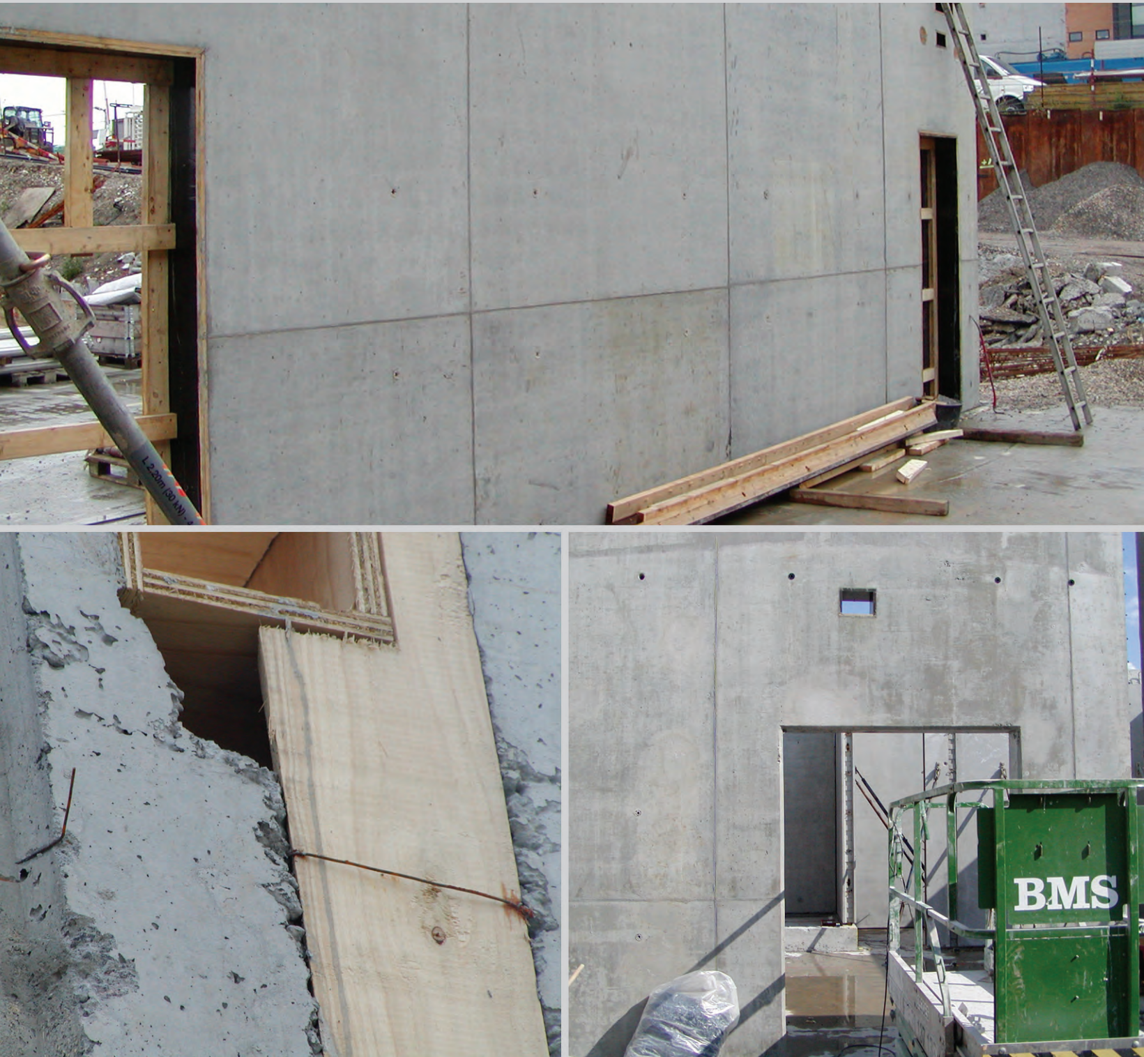
Figure 2.6. Examples of form filling with SCC. Top right and bottom right are examples of complete form filling. SCC closes around all boxouts and flows out into all corners. Bottom left shows an example of incomplete form filling with honeycombing and holes below a boxout.
