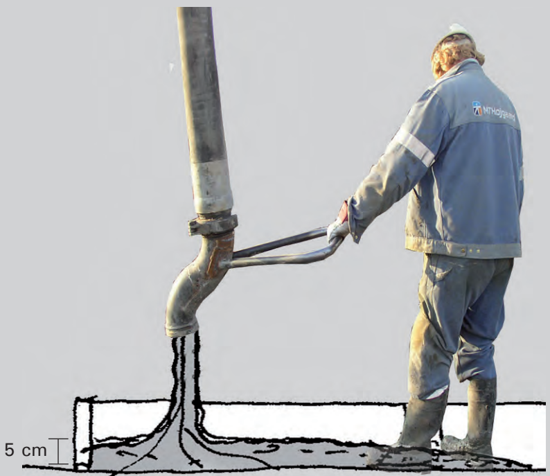
Figure 4.4. Example of floor casting with a high slump flow value of approximately 675 mm. Poor control of the concrete front, flowing a rather long distance from the inlet. It is not possible to achieve a final concrete slab depth (e.g. 100 mm) during a single filling process as the concrete will flow up to 4 m away from the inlet. This contributes significantly to an increased risk of dynamic segregation. It is not possible to cast the concrete floor without having to walk in the concrete.
