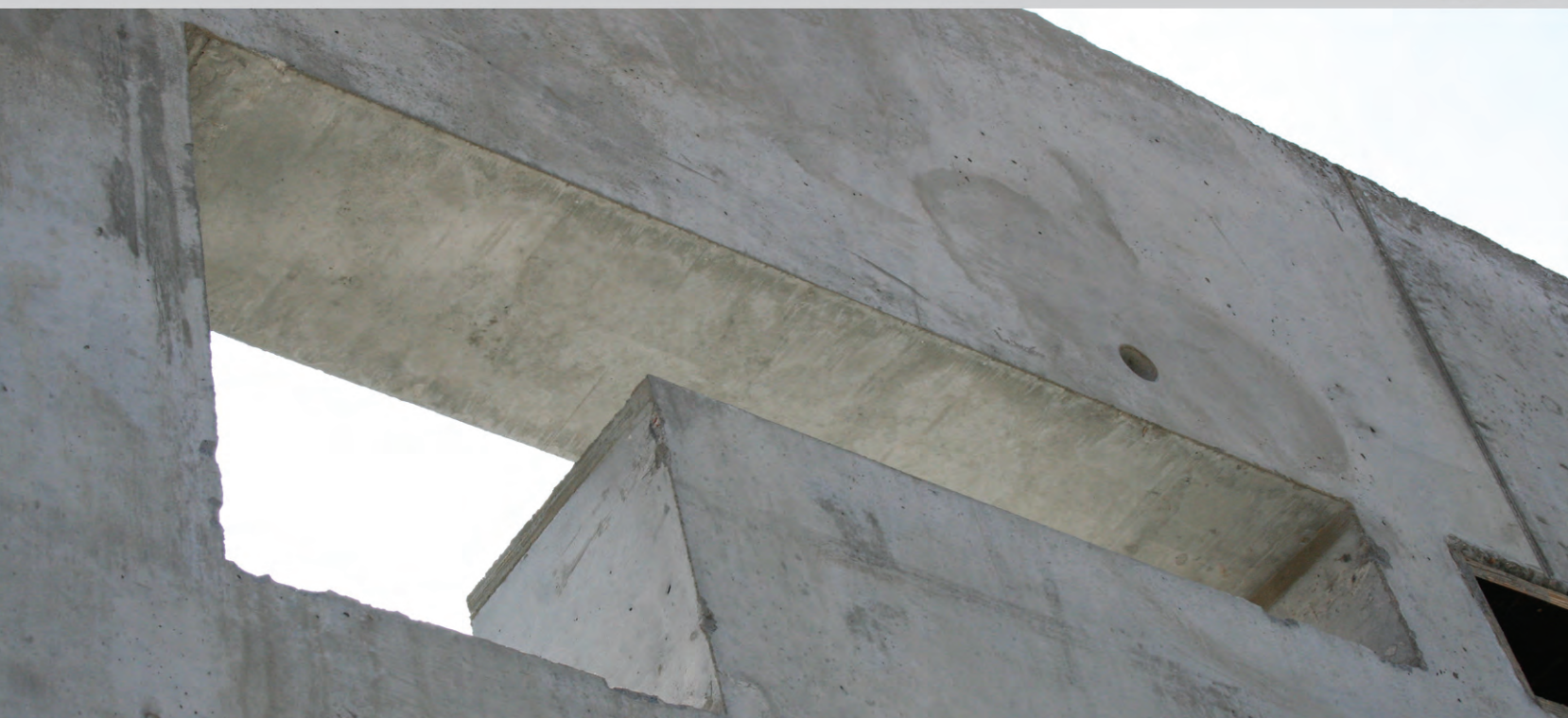
Figure 2.7. Example of complete form filling, where the SCC closes around the L-shaped boxout, flowing into all corners. In this case casting with SCC has saved the planning and execution of access channels for poker vibrators.
