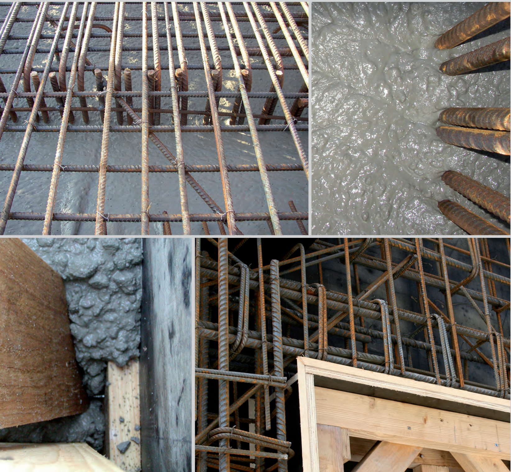
Figure 2.13. Example of no blocking. SCC flows well around the reinforcement without accumulation of aggregates.
