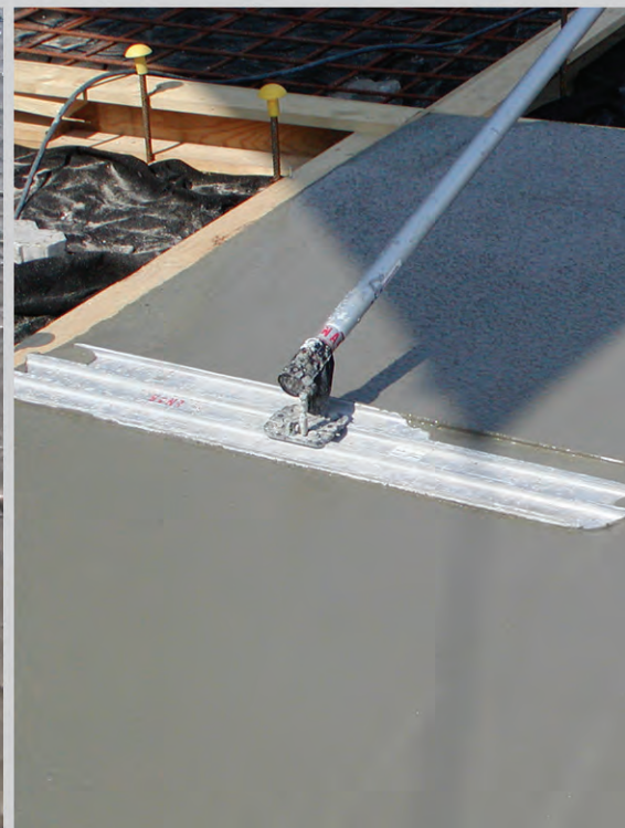
Figure 4.6. Upper right: Curing membrane is sprayed on as soon as the surface is levelled. This should be done as soon as possible after the surface finishing process. Upper left: Visible coarse aggregates in the surface are submerged with a piece of drainpipe mounted on a shaft. Bottom right: The surface is levelled with a surface planer tool. It is not recommended to use the planer when there is a large number of coarse aggregates in the surface as they may leave tracks in the surface. Bottom centre: SCC where segregation has clearly occurred. There are no visible aggregates in the surface or just below it. The surface is also bubbling due to instable air voids. Bottom left: SCC without segregation having visible aggregates in the surface.
