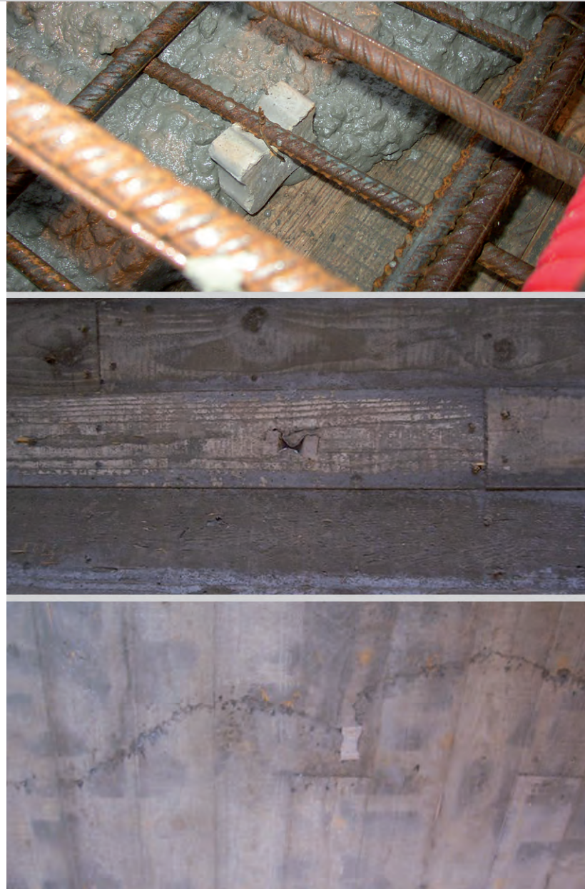
Figure 2.14. Top: Spacer is being embedded by SCC. Bottom and center: Visible tracks and footprints from the spacer in bridge deck soffit.
