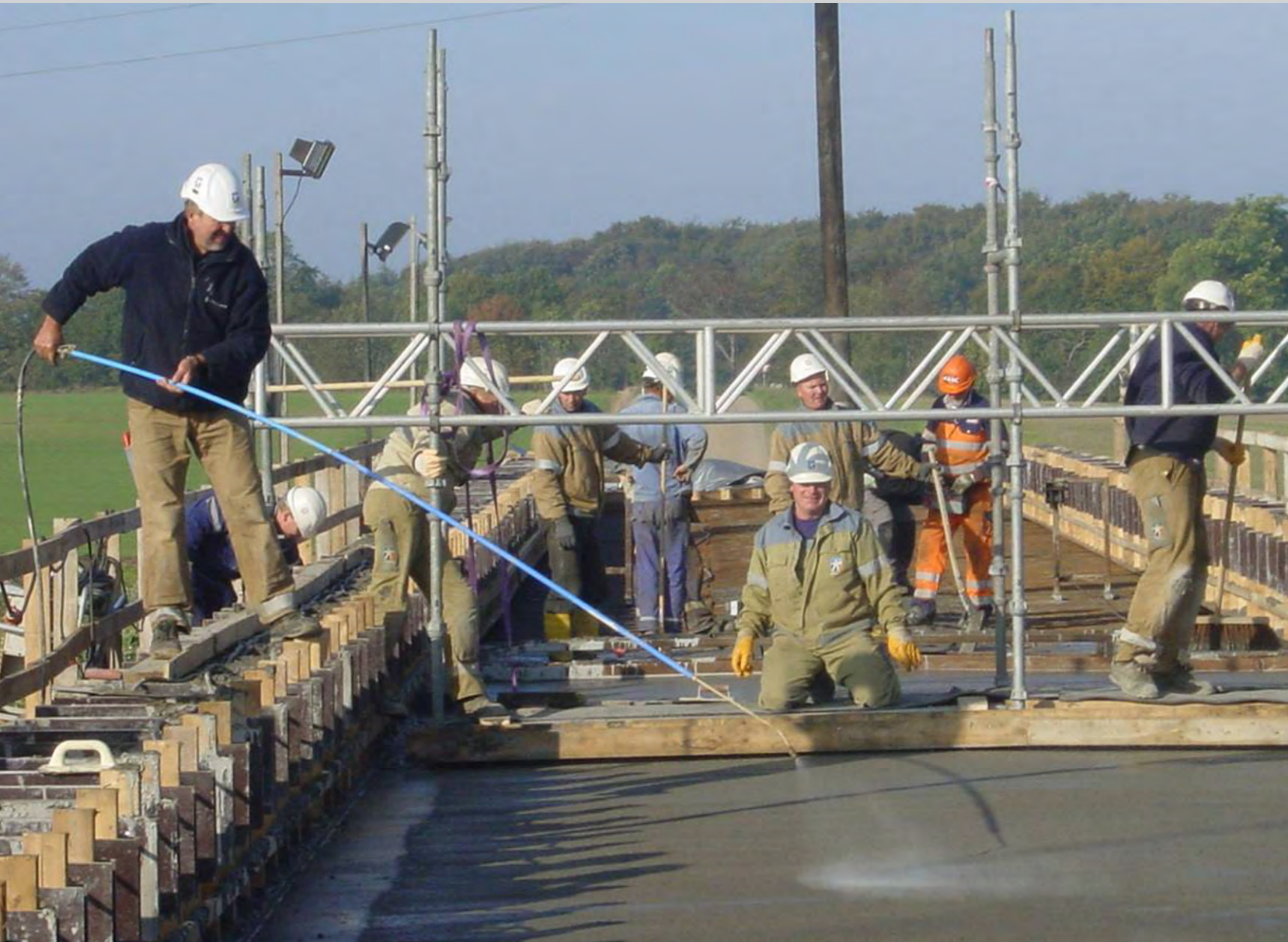
Figure 2.16. Application of curing membrane to an SCC bridge deck as a temporary protection measure, followed by plastic covering as shown in Figure 2.15.
