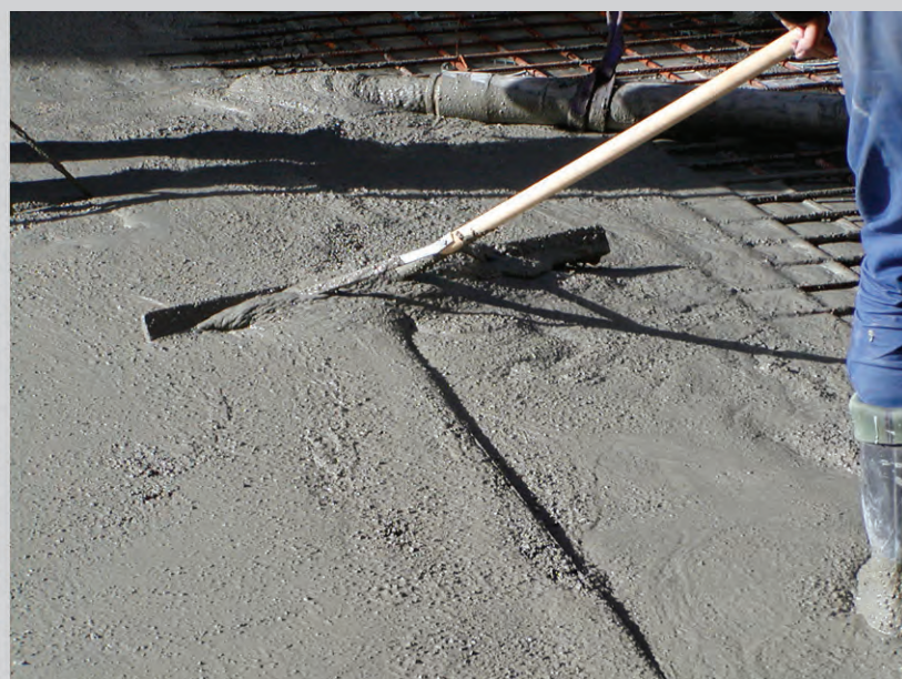
Figure 4.5. Left: Horizontal casting of SCC. Right: SCC is placed using a scraper so that the concrete is redistributed in order to obtain correct slab thickness.
