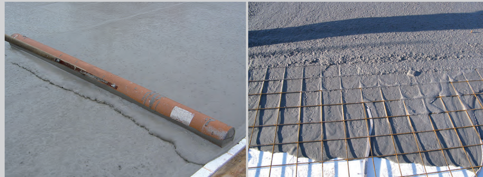
Figure 2.8. Segregation during horizontal floor castings.
