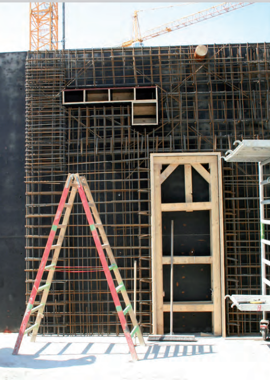
Figure 2.3. Preparations of wall formwork with a height of approximately 4 m. Example of recesses and box outs.
