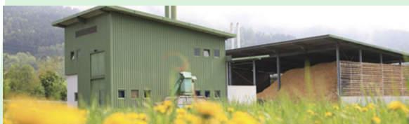
Figure 3: District heating plant in Austria. The wood chips storage is located to the right, and the boiler house to the left.
