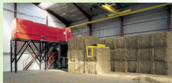
Figure 4. The automatic crane is in waiting position, until the control system "calls" for straw. The crane lifts the bale up to the straw shredder where the gate opens automatically. The bale is shredded and screwed or stoked into the boiler
