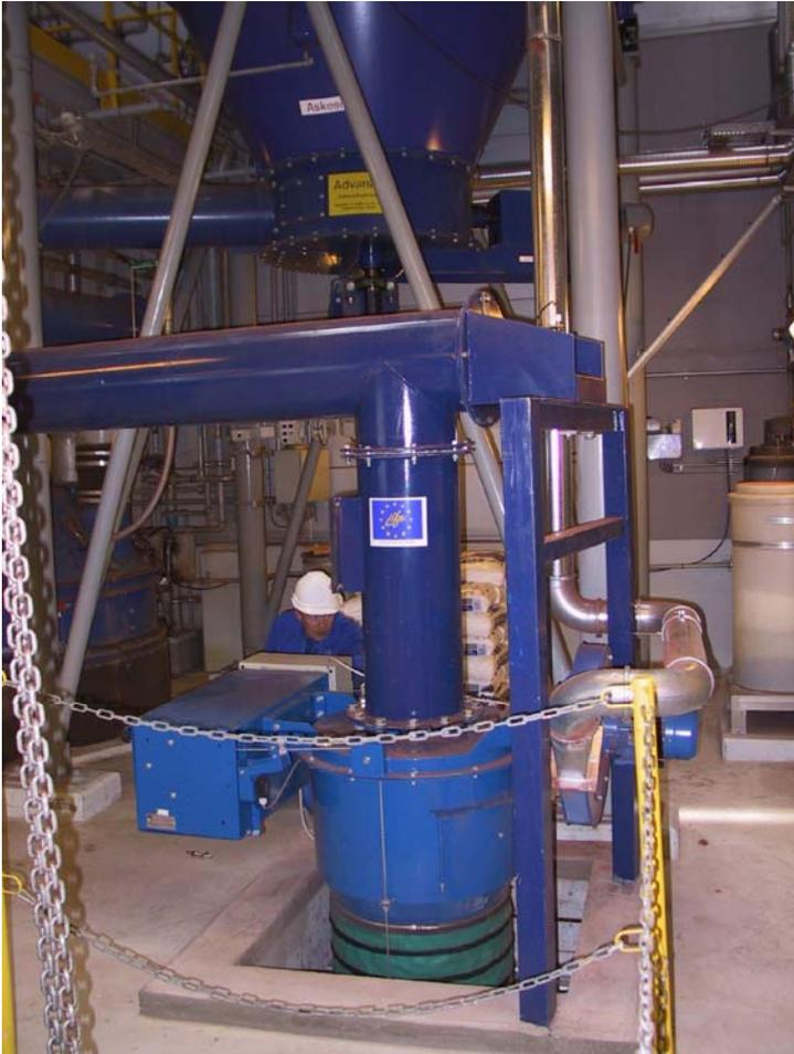
*Figure 2. The new dry ash outlet at AWS with screw conveyor and load bellows.*
