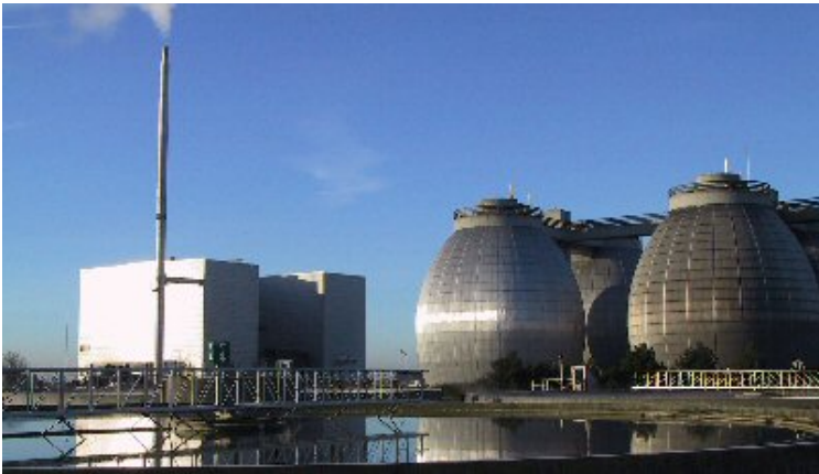
Incineration plant and aerobic digester at Avedøre Wastewater Services.
