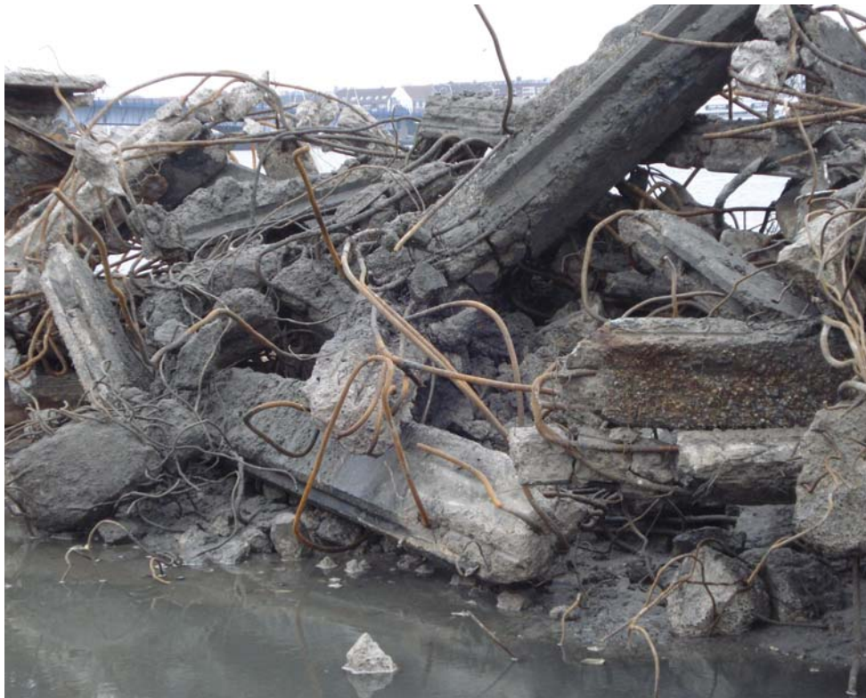
Figure 2. Construction and demolition waste may need extensive and costly sorting before it is ready for secondary use.
