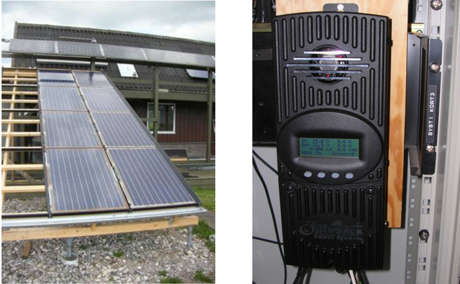
Fig. 25. PV array with 2 x 4 modules in series and MPP charge regulator
