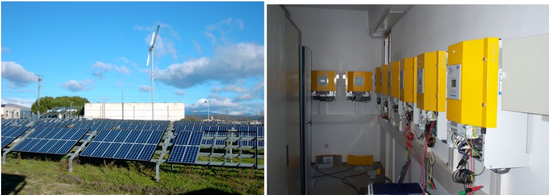
Fig.5 Hybrid 3 phase AC system with SMA inverters (Spain)
