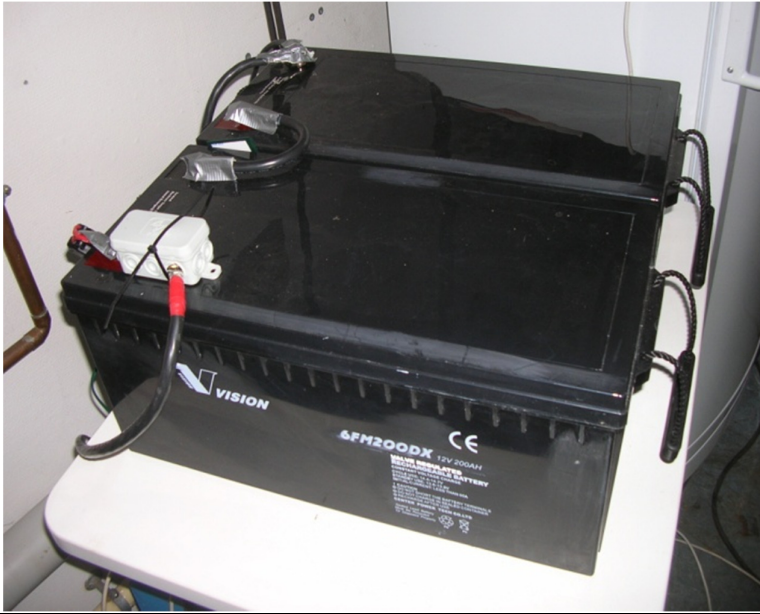
Fig. 27. Battery pack with two AGM sealed lead-acid batteries
