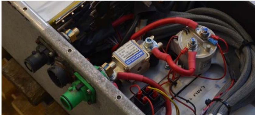
Figure 3.1.19: Fuse and Contactor relay in rear battery box
