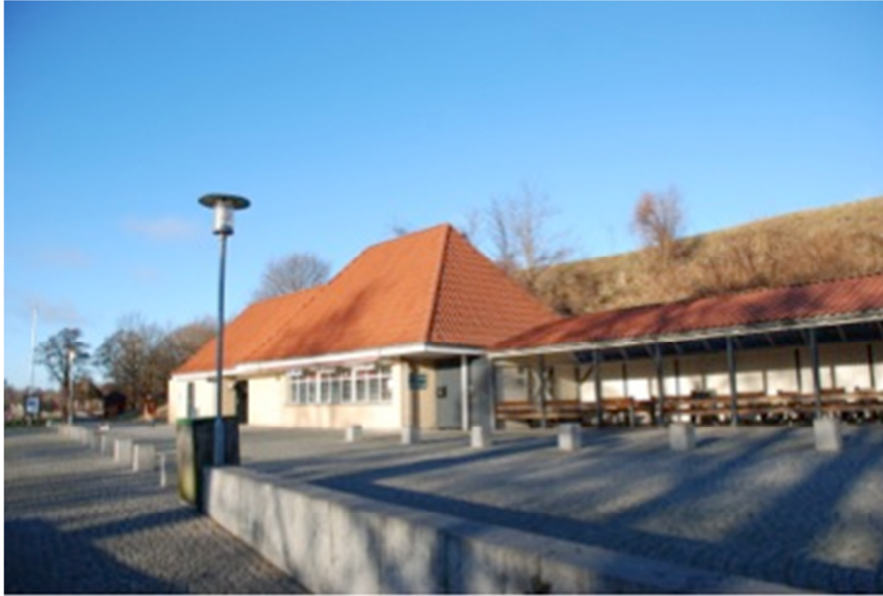
Figur 18 Kiosk and toilets at Ry Harbour
