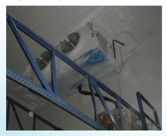
Huge energy losses Temperature rise in the cold sections Ice on the refrigeration units Ice on the floor
