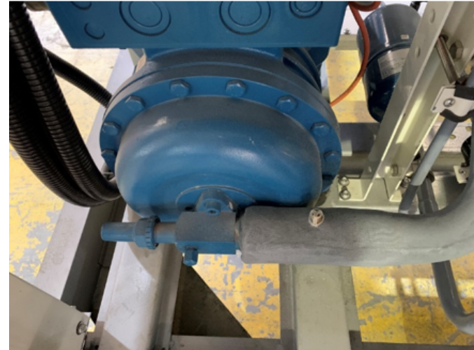
Compressor Suction Shut Off Valve
