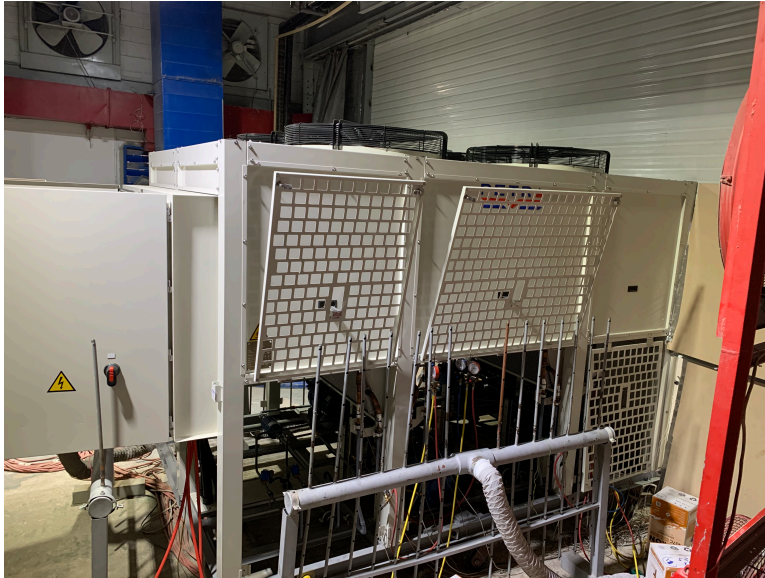
Rooftop Package unit – condenser side
