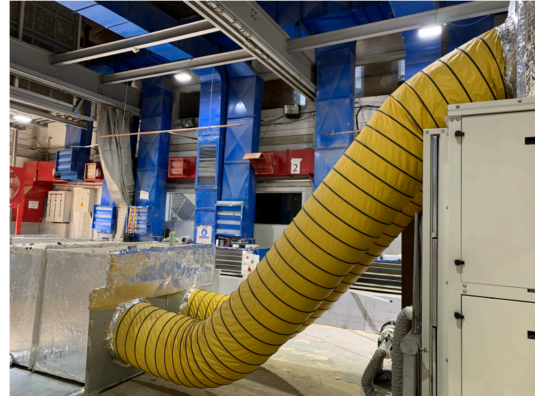
Rooftop Package unit – AHU side
