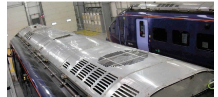
Example rail AC unit mounted on top of passenger cars
