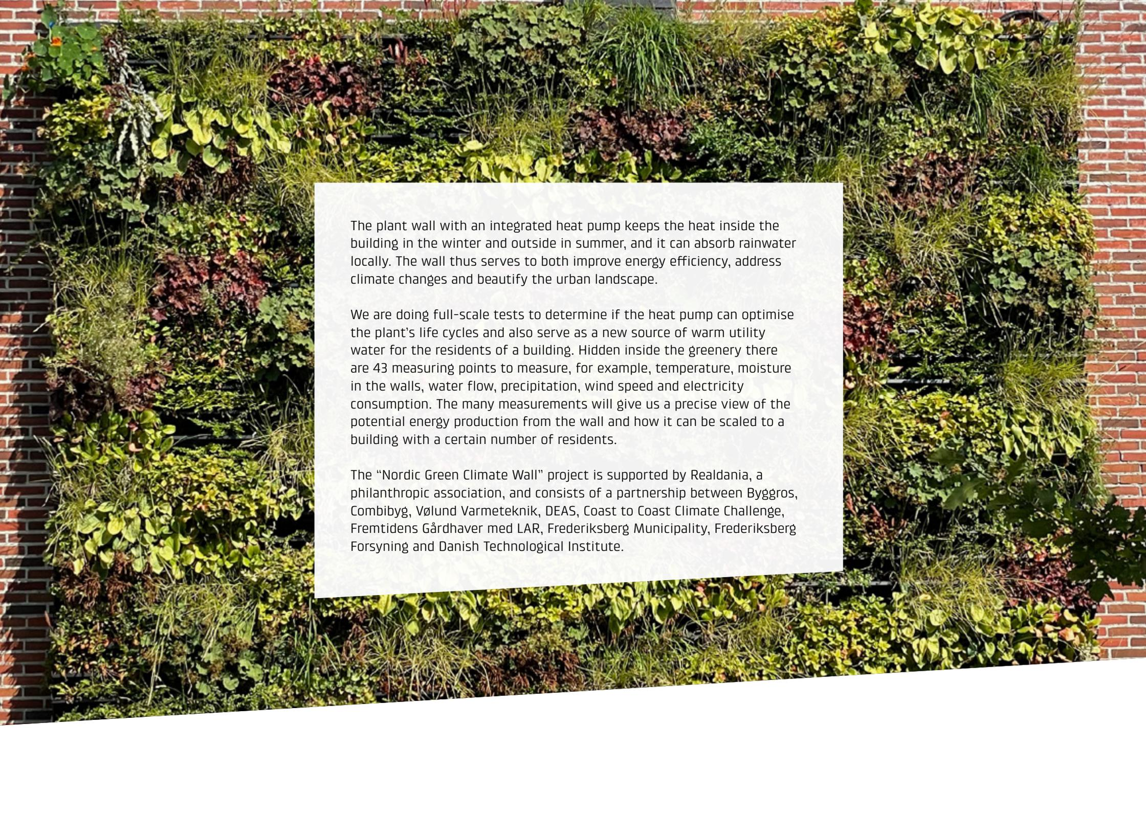
The plant wall with an integrated heat pump keeps the heat inside the building in the winter and outside in summer, and it can absorb rainwater locally. The wall thus serves to both improve energy efficiency, address climate changes and beautify the urban landscape.
