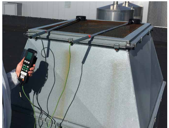
On-site air flow measurements
