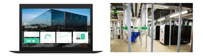
Figure 73: EMV dashboard with quick overview of current performance (left) and an Energy Machines heat pump installation with sensors placed inside the boxes (right).
