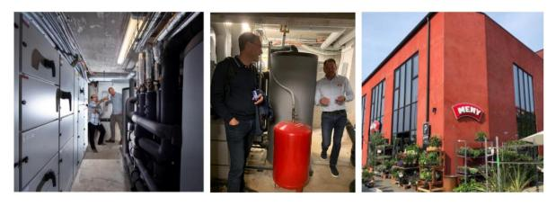
Figure 62: Heat is recovered from a supermarket refrigeration system to the local district heating grid in Copenhagen.
